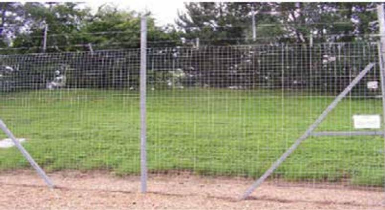
A Class 2 Anti Intruder fence 2.9 metres high constructed with welded mesh fabric and topped with barbed wire systems.
