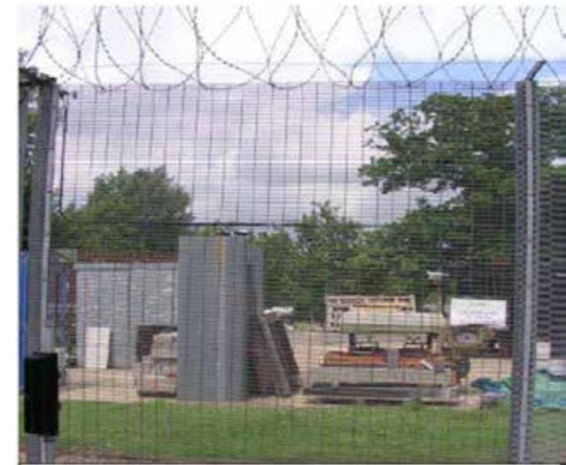
A Class 3 welded mesh fence which complies with BS 1722 part 14. The fence is 4 metres in height, and is constructed using narrow aperture welded mesh to resist climbing and cutting and is topped with barbed tape/razor wire concertina.
