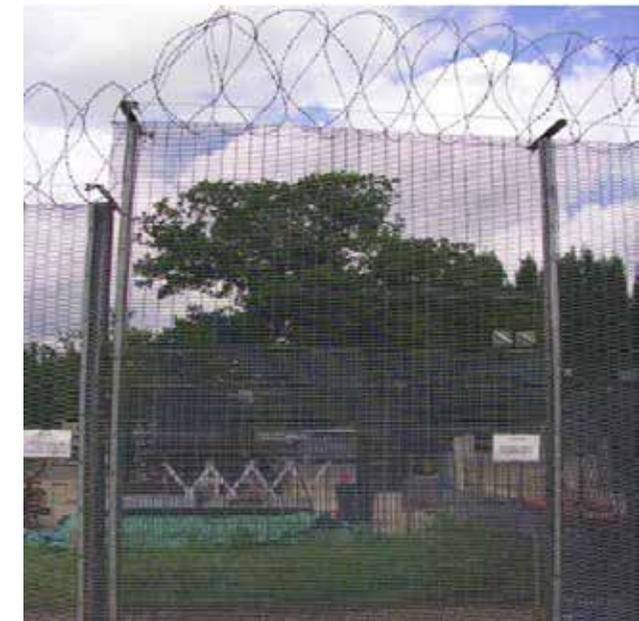
A Class 4 high security welded mesh fence to BS1722 Part 14 standard. It is 4.8 metres high including barbed tape/ razor wire topping. It is constructed using narrow aperture welded mesh with an additional layer up to 3 metres in height.
