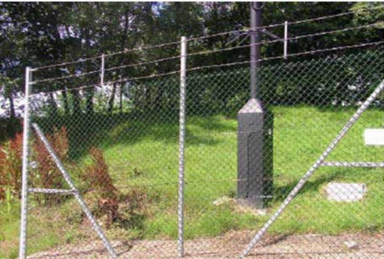
A Class 1 chain linked fence height 2.9 metres high, constructed with chain link fabric and topped with barbed wire topping. The supporting posts are either of reinforced concrete or tubular steel
